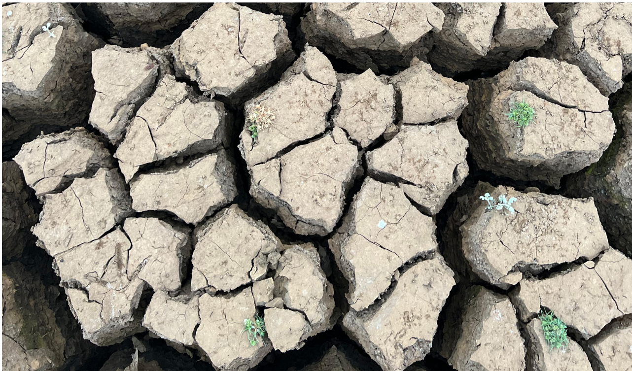
The dry bed of a silted dam: where stored water should have been, only cracked earth remained.
